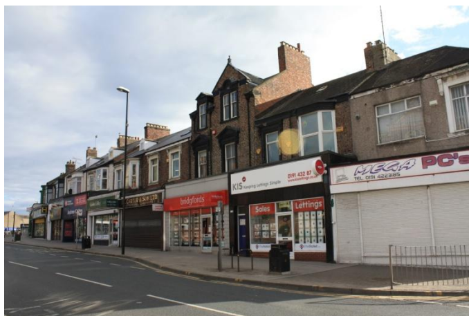
Photograph 7—Buildings along Fowler Street
