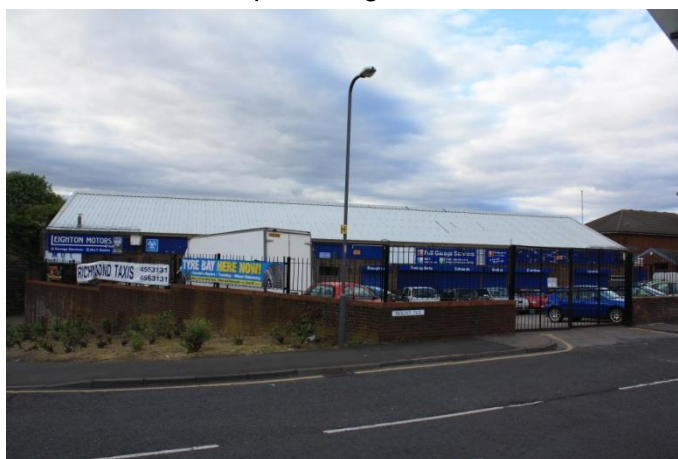
Photograph 6—Car workshops on Mount terrace with corrugated metal roof
